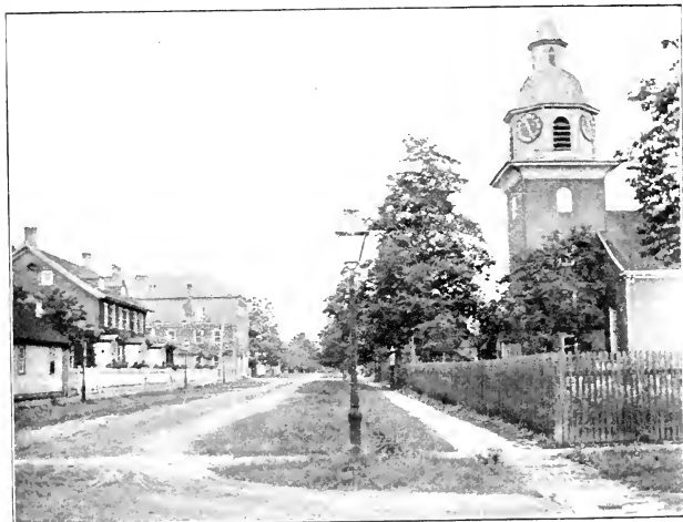
Street in Economy, showing the Church, Town Hall and "Great House."
